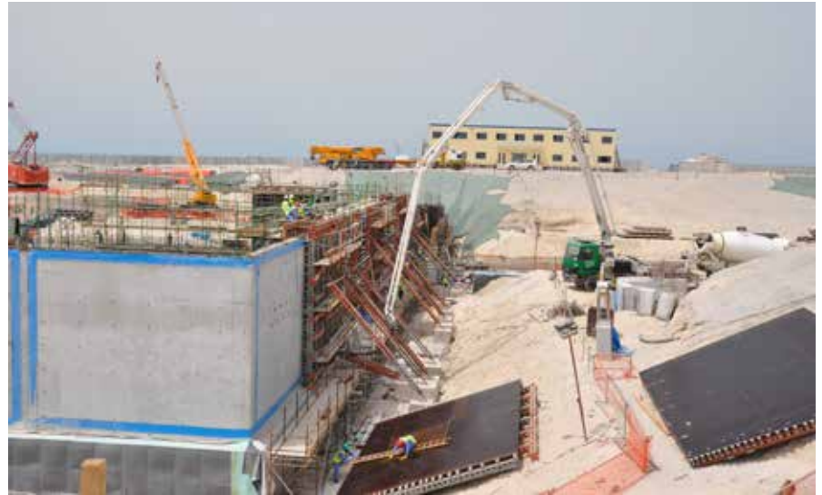
Figure 2: Concrete pump connected to the bottom side of the formwork
