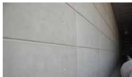
Figure 8: final surface finish of the Performance Engineered Concrete
