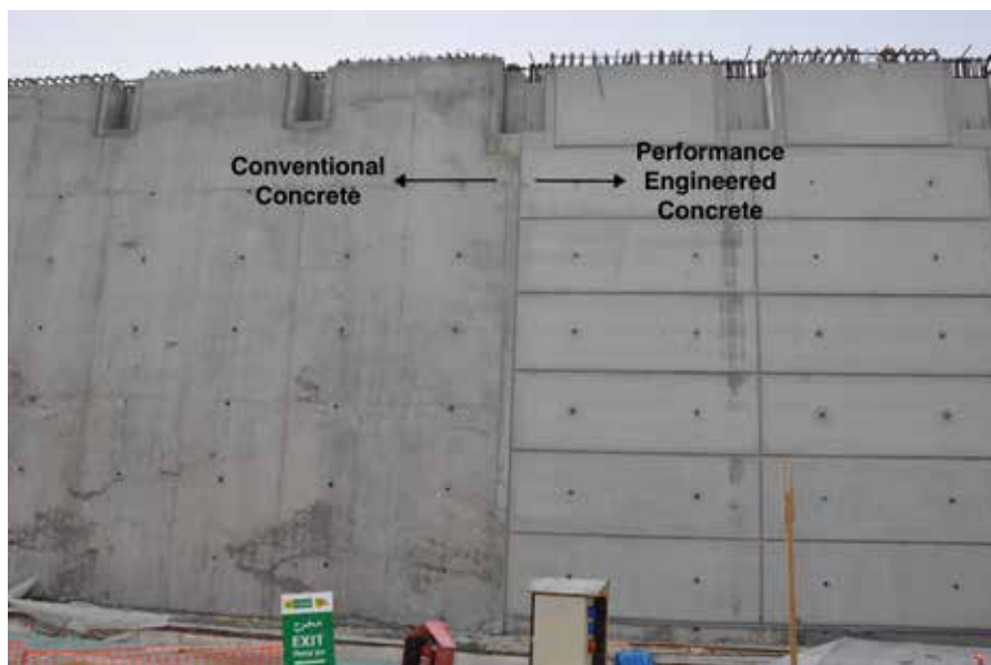
Figure 6: Conventional vs Performance Engineered Concrete - mockup
