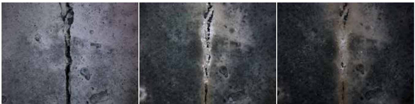
Figure 3. Healing of 0.8 mm wide crack in concrete specimen amended with powder compressed healing agent. Left picture: freshly cracked specimen; middle picture: same specimen after 28 submersion in water; right picture: same specimen after 56 days submersion in water. Image courtesy of Renee Mors.
